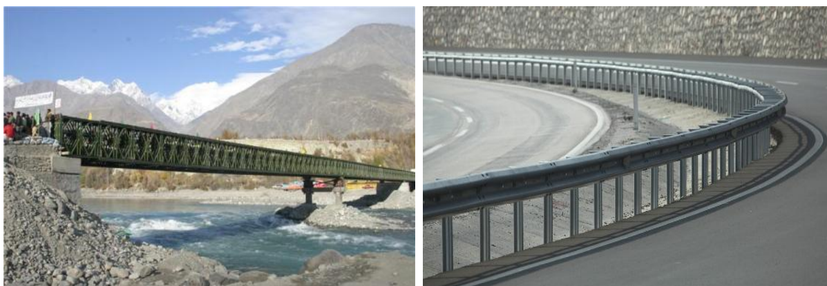
Figure 22: Steel Bridges (Left) and Steel Crash Barriers (Right)
