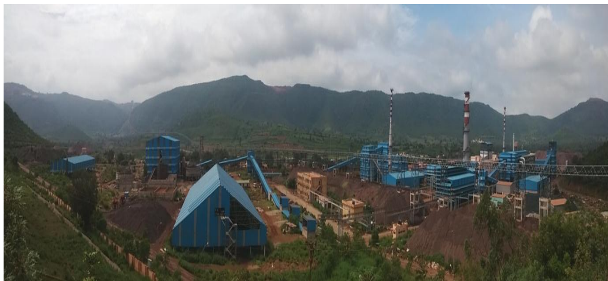
Figure 39: NMDC's new pellet plant in Donimalai, Karnataka
