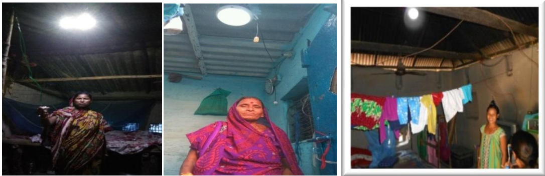
Surya Jyoti installed in rural houses and urban slums
